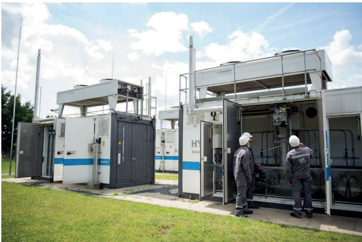
Figuur 23: AEL Elektrolyse (Hydrogenics) Falkenhagen Germany
